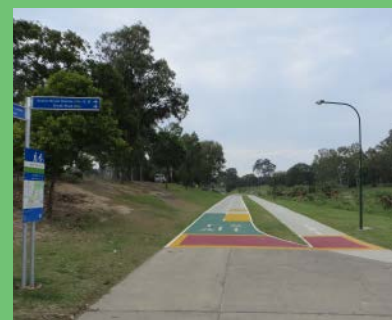
Kedron Brook Bikeway on Brisbane's north side which duplicates an existing narrow shared path to provide separated pedestrian and cycling facilities.
