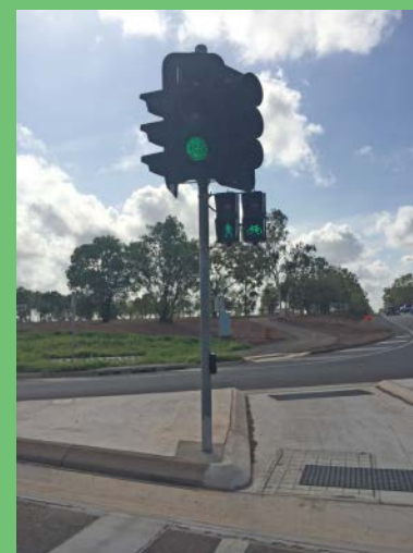
An intersection on the Stuart Highway in Darwin was upgraded to provide a signalised crossing for pedestrians and bicycles.
