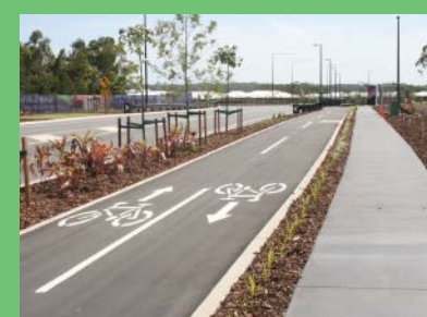
New greenfields sites in Caloundra South, Queensland have been provided with fully-separated bicycle paths and pedestrian paths.
