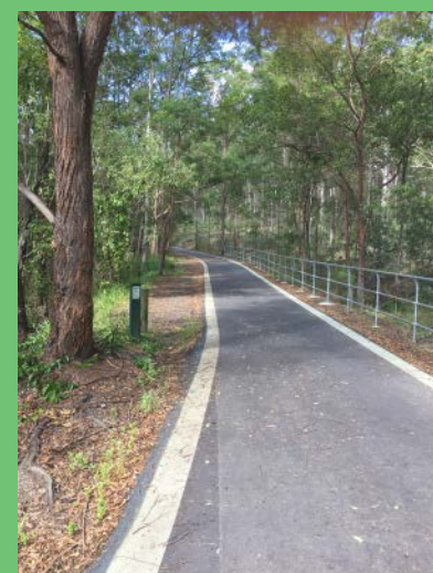
Stage 1 of the Samford to Ferny Grove cycle link. This path follows the route of a former railway line.
